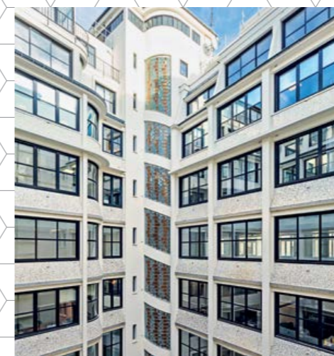
Renovation of 9 Percier.
